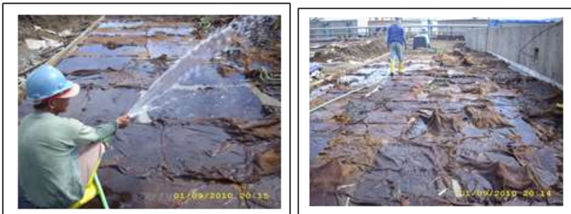
Gambar 2.1 Perawatan beton ( water curing )
