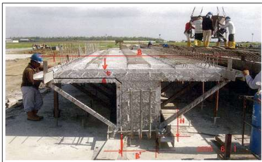
Gambar 2.23 Beton Precast T
