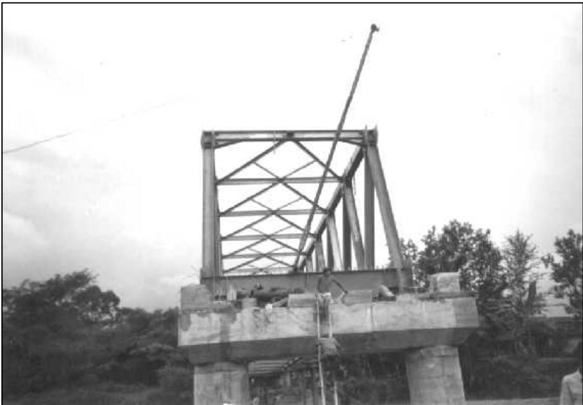
**Gambar No.18.b: Tiang Crane Sederhana**
