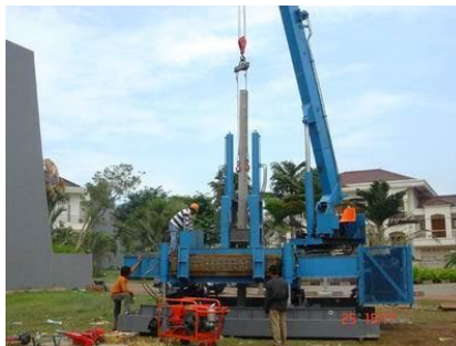
Gambar 2.12 Hydraulic static pile driver
