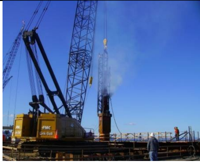
Gambar 2.11 Diesel Hammer
