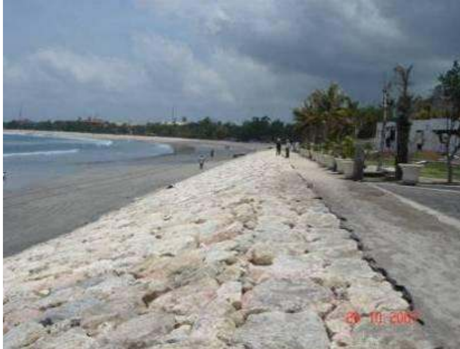
Photo 3 Bangunan Pengaman Pantai - Revetmen
