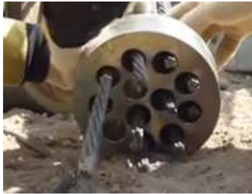
Gambar 4. 7. Pemasangan wedges multi use/ wedges plate
