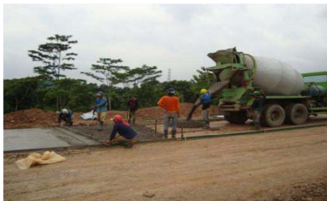
Gambar: Truck mixer sedang menghampar beton Lean concrete
