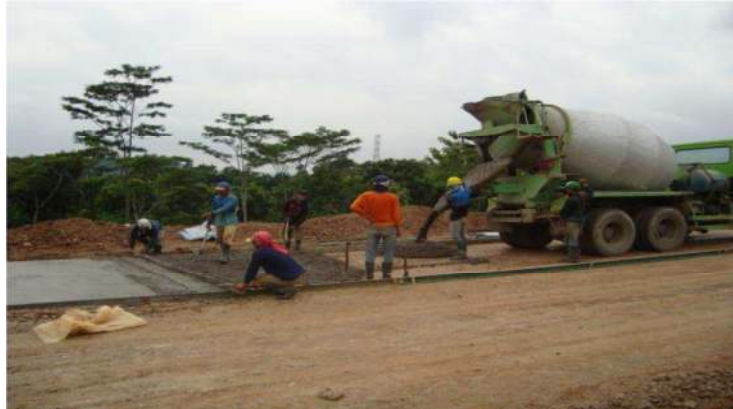
Gambar 16 : Truck mixer sedang menghampar beton Lean concrete
