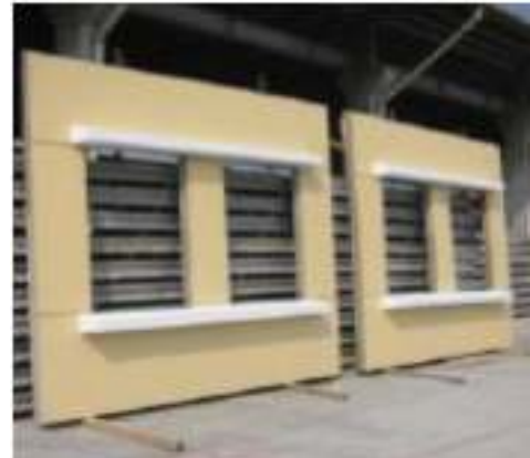
Gambar 4.4 Dinding Precast
