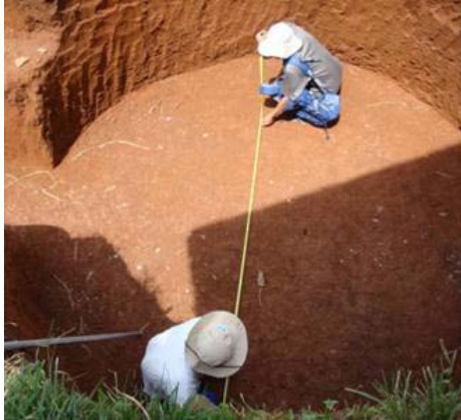
Gbr 4.138 Memeriksa diameter lubang galian
